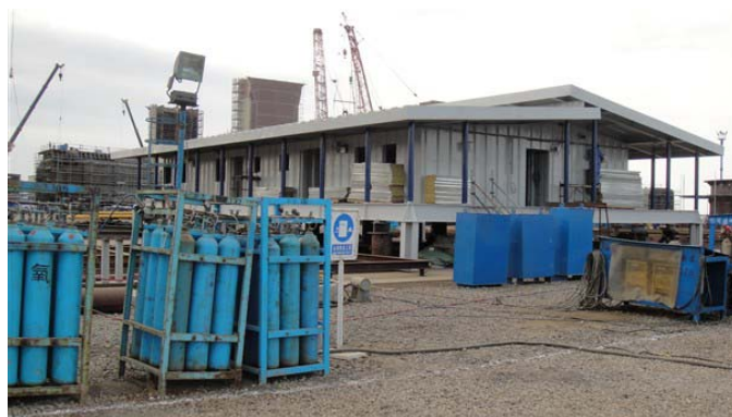
CONTROL BUILDING 外部结构
