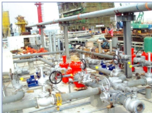
平台工艺管线组装 Assembling platform process piping
