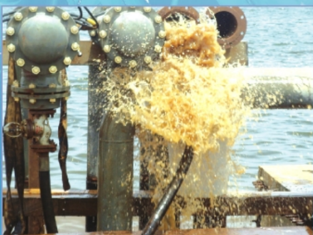
清管试压 Pigging and Hydro test
