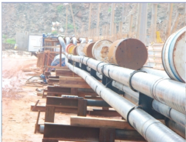
绑扎好的管线和浮筒 Pipeline Bundle and Buoys
