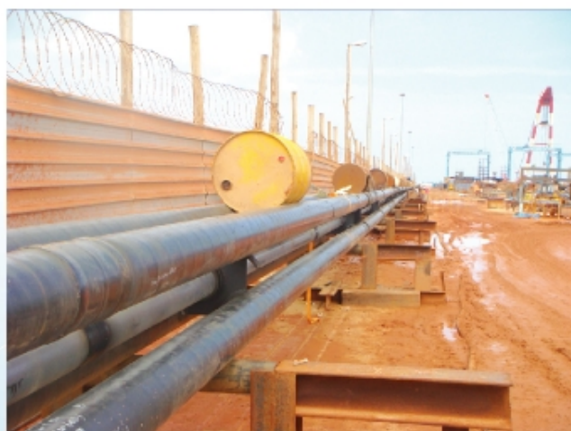
绑扎好的管线和浮筒 Pipeline Bundle and Buoys
